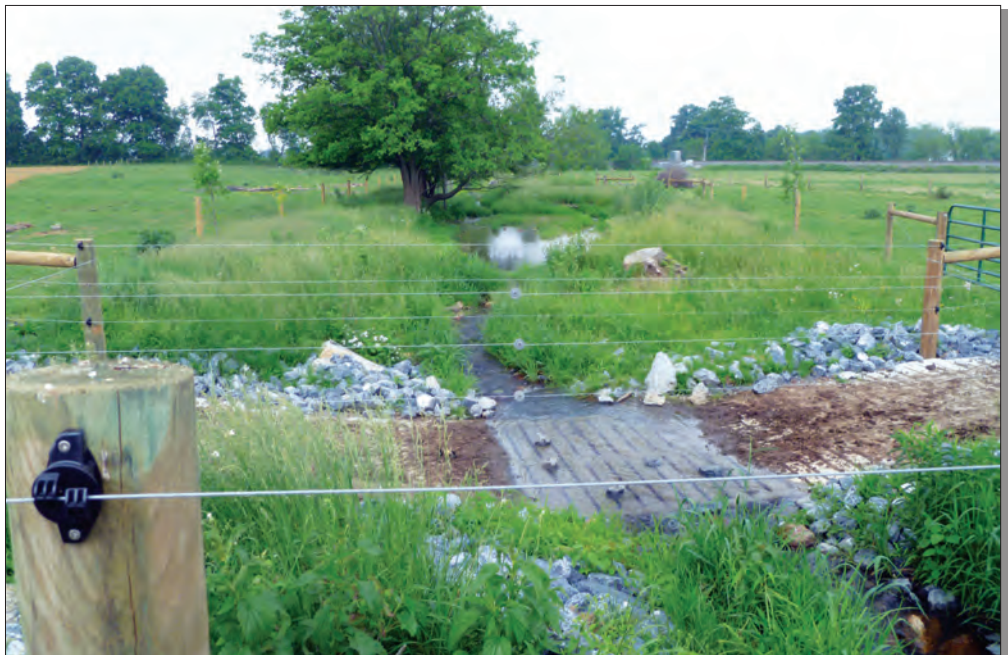
Stream crossings help improve water quality by limiting livestock access and protecting stream banks.
