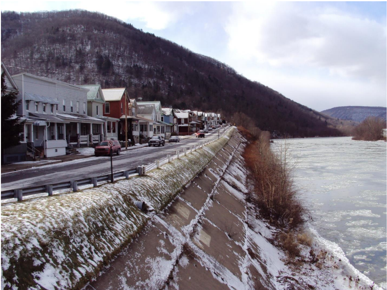
Riverview homes in South Renovo
