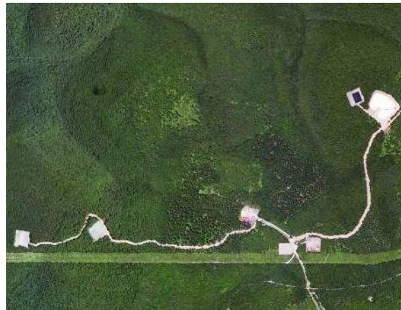
Array of well pads alongside a transmission corridor
