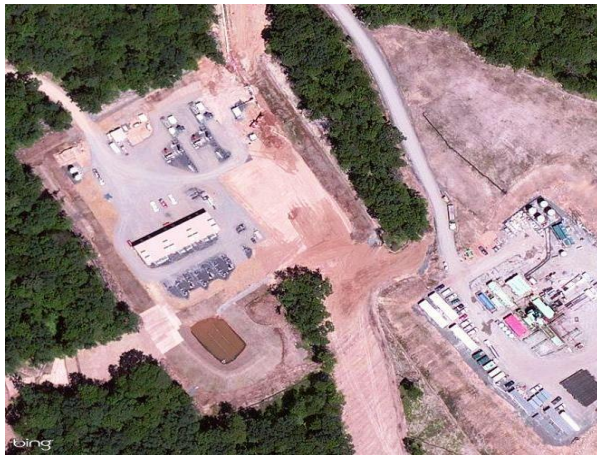
A compressor station (left) near a well pad (right)
