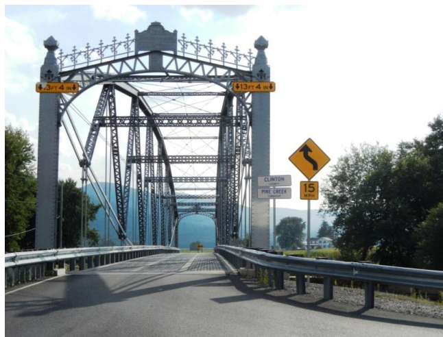
Pine Creek Bridge, Pine Creek Township
