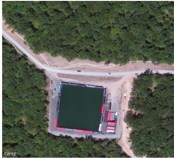
A water impoundment with piping
