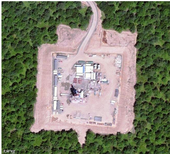
Well pad with drill rig in place
