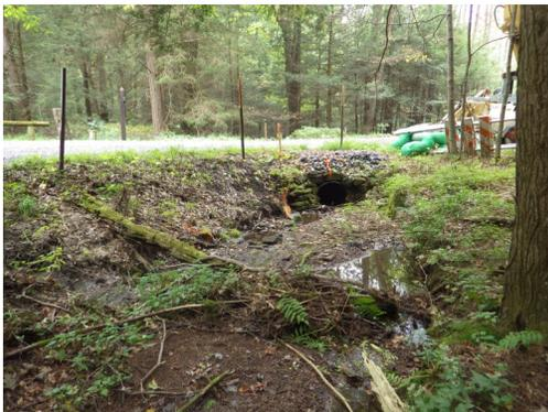
**AFTER:** An aluminum arch structure with a full plate bottom was constructed at “bankfull” width of the stream (9’) in order to accommodate high flows and restore the stream corridor.
