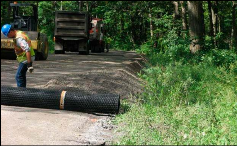
Use pervious surfaces on sites where there is no threat of contaminated runoff.
