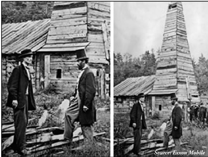
The first successful oil well was drilled in Titusville, PA.
