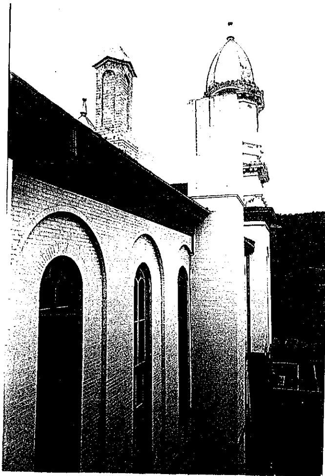
(12) View of chimneys at east elevation.
