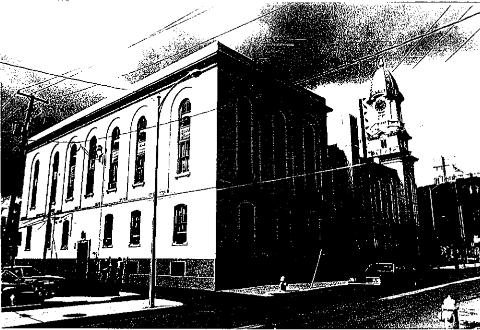
(4) View looking northwest at the south entrance.
