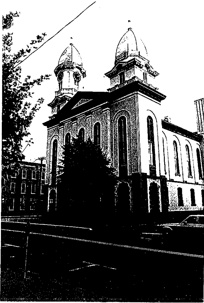
(3) View looking southwest at the main entrance to the building.
