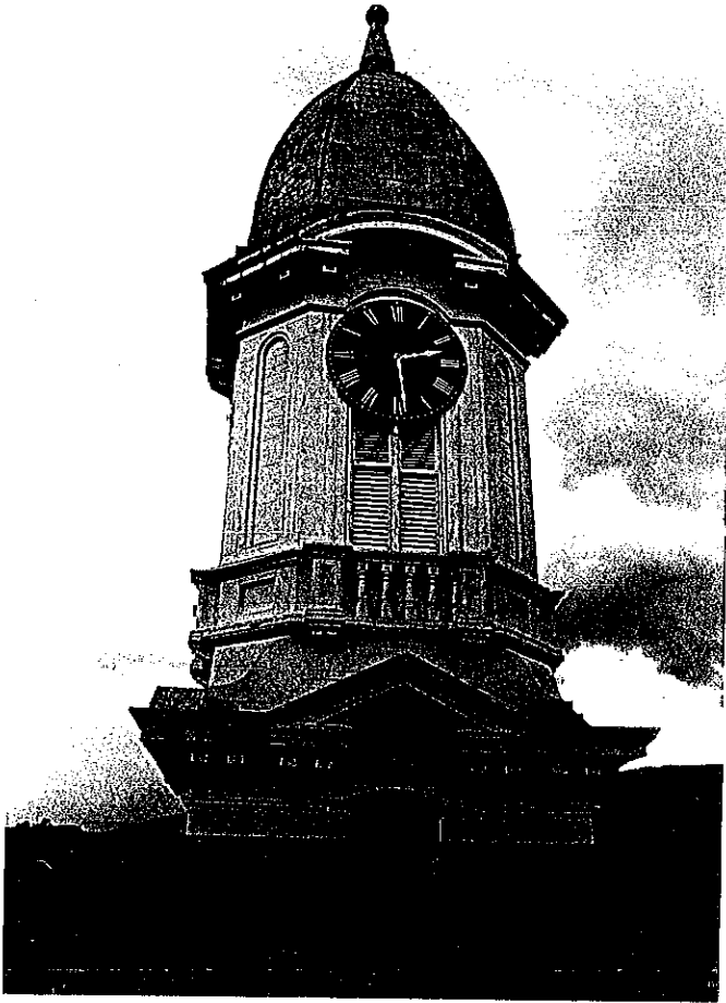
(5) View of the western face of the clock tower.
