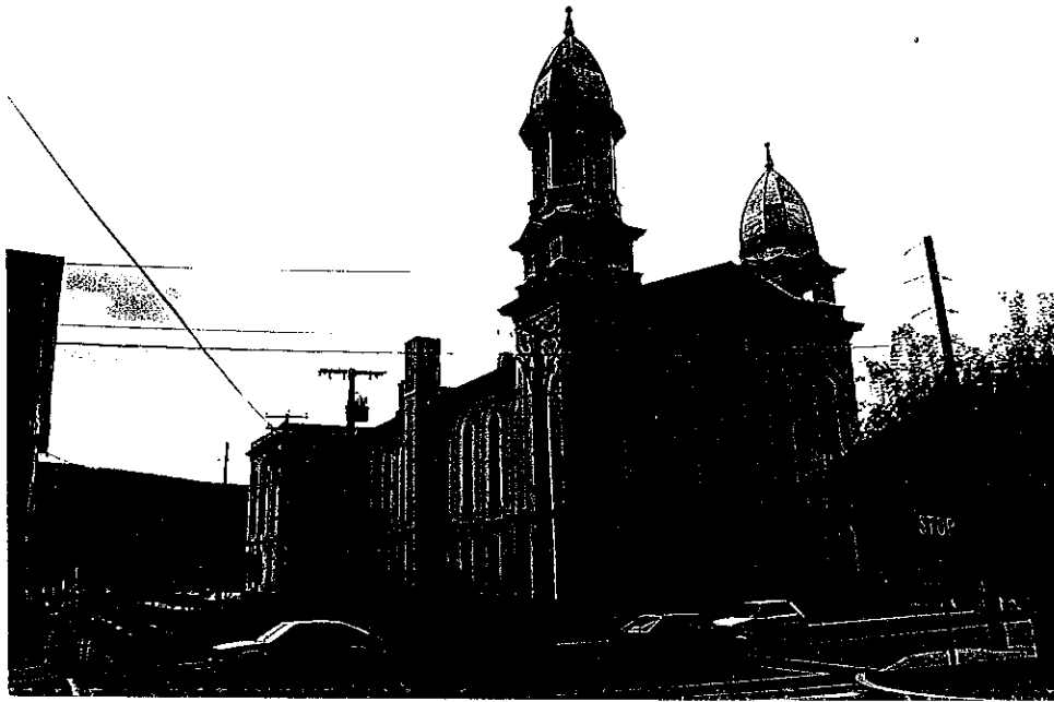
(1) View looking southwest at the north entrance to the building.
